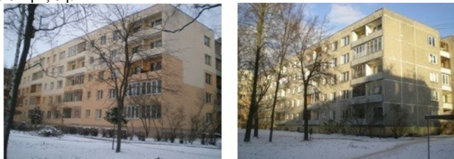
Fig. 5 Typical dwelling house in Latvia (Series 464) – before and after renovation
