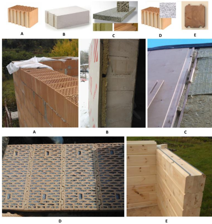
Fig. 3 Exterior wall base construction materials and construction process (type A, B, C, D, E)
