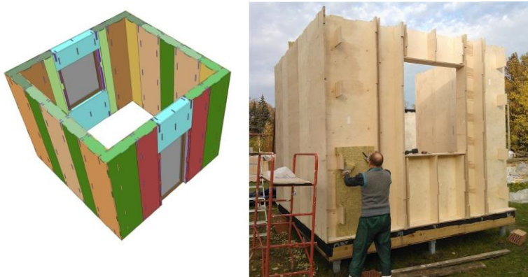
Fig. 4 Plywood frame structure installation design (type C)
